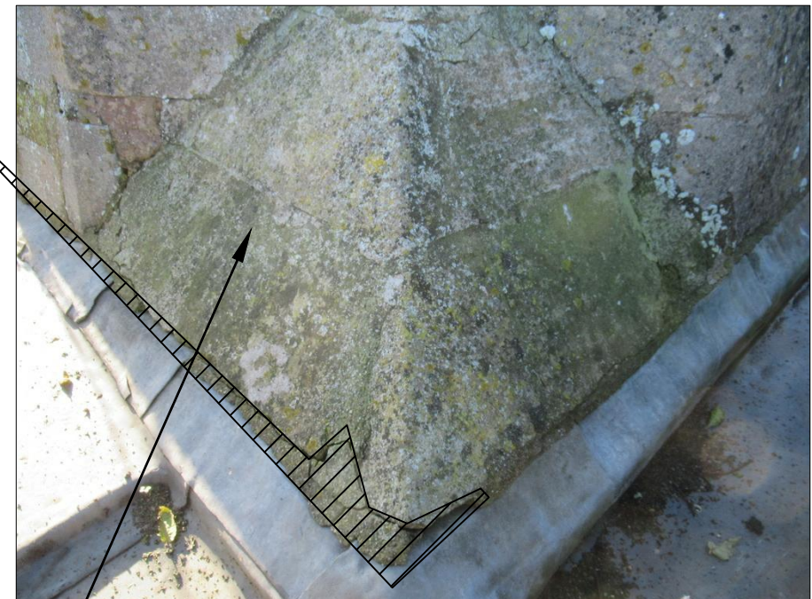
TOWER - NORTH EAST BROACH
