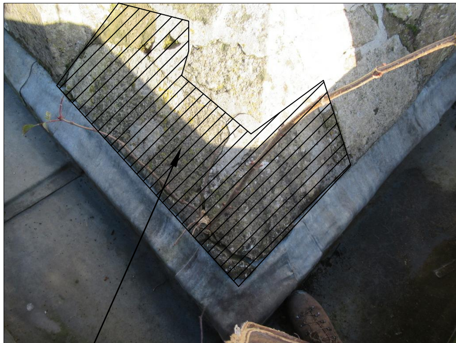
TOWER - SOUTH WEST BROACH
