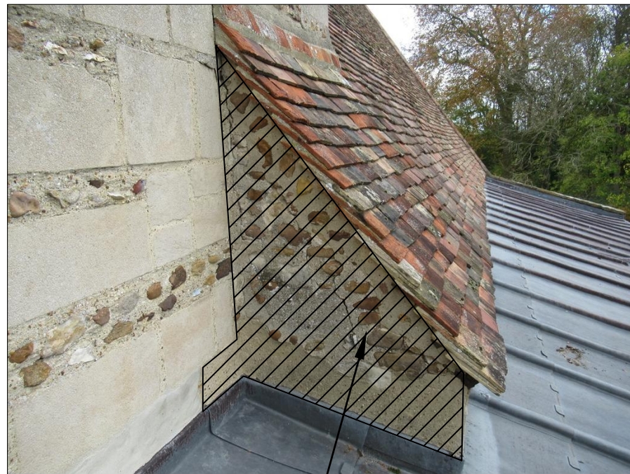
SOUTH AISLE ROOF - SPANDREL WALL PANEL
